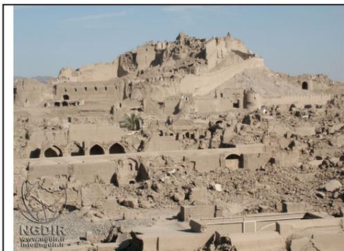
**Figure 1:** Damage in the old city of Bam due to the M6.6 earthquake of 26 December 2003. The fatalities numbered 22,500, which was about 1/3 of the population, an unusually high rate due to the poor construction. Rapid mobilization of rescue efforts is important because injured trapped beneath the rubble can be rescued alive for a few days only.
